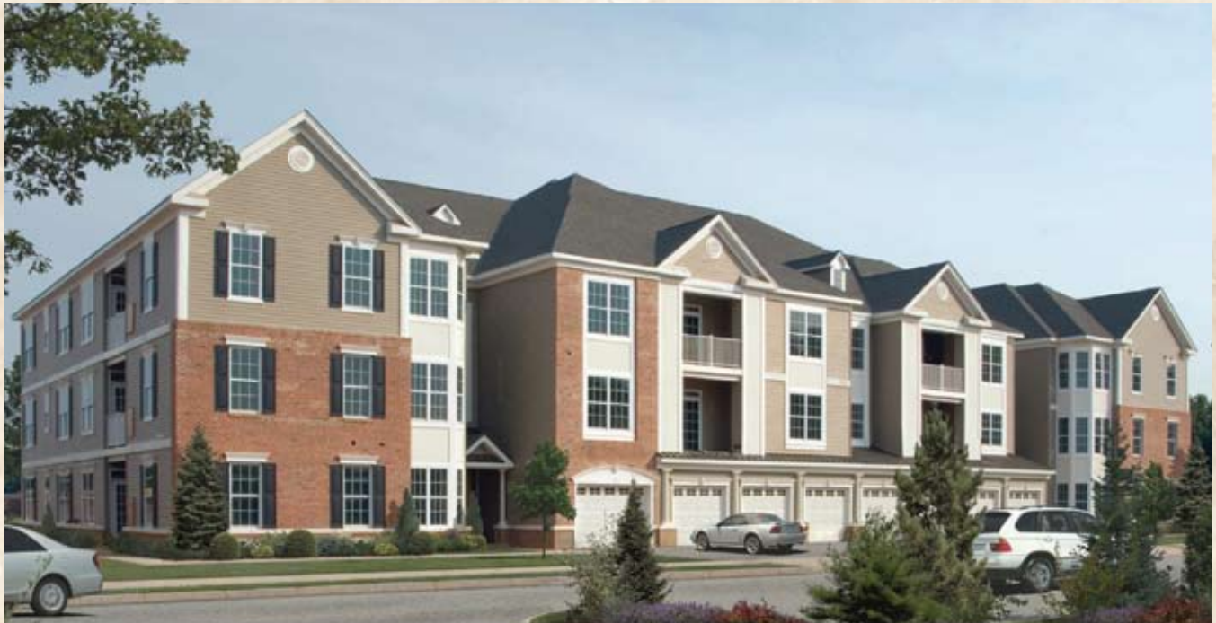
The Lennar Centre Place at Edison is a redevelopment of a former military arsenal in Edison, New Jersey.
